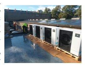
London) and four 11kWp air source heat pumps on its roof. The system is supported by three 13.5kWh batteries, enabling the church to be completely off-grid for many months of the year. Stokey Energy worked closely with Alex Sheratt, a senior architect and member of the congregation, to ensure that planning was secured from both the local authority and the Diocese of London, while grants from the London Legacy Development Corporation and Hackney Light and Power helped make it possible.
